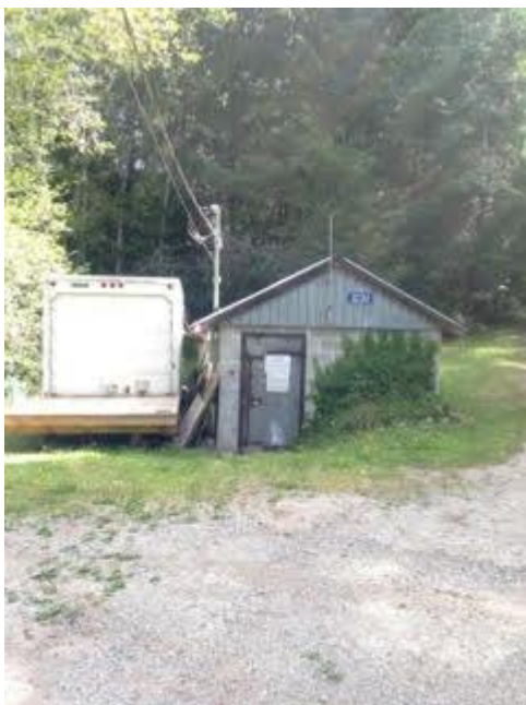
Main Pump House – Located at 9730 Emil Road, Lund, BC
